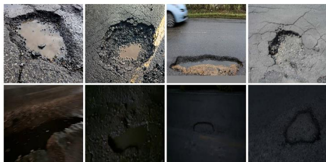
Fig. 5 To illustrate robustness of the two modal approach, Fig 5 shows that when the visual approach is not possible due to darkness or shadows, the data from the inertial sensors agrees with the pothole's existence.
